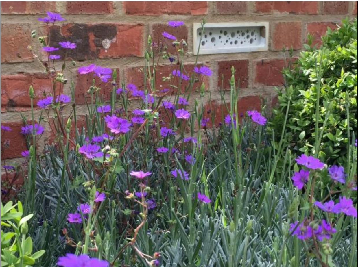
Figure 7-1: Example of an installed bee brick (Green & Blue, 2026)
