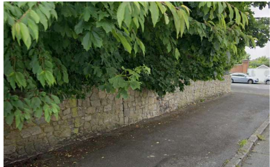
Plate 4: Northern boundary wall for overgrown area in northwest, facing west
