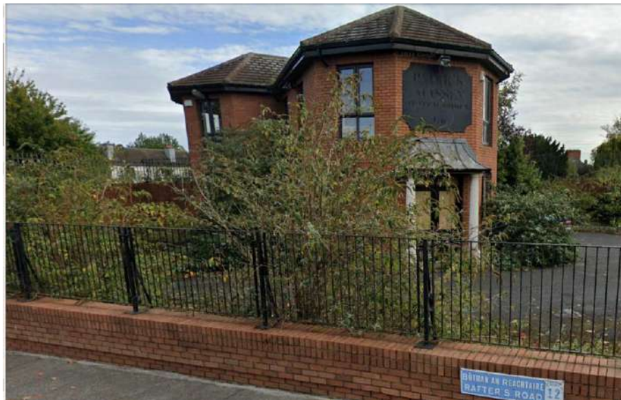
Plate 3: Former funeral home on Crumlin Road/Rafter's Road, facing northeast
