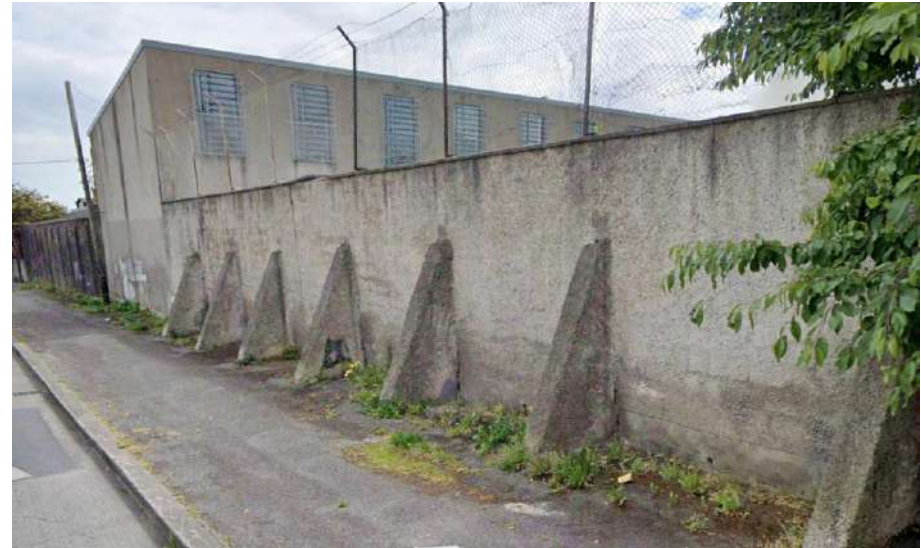
Plate 2: Northern boundary wall, facing east
