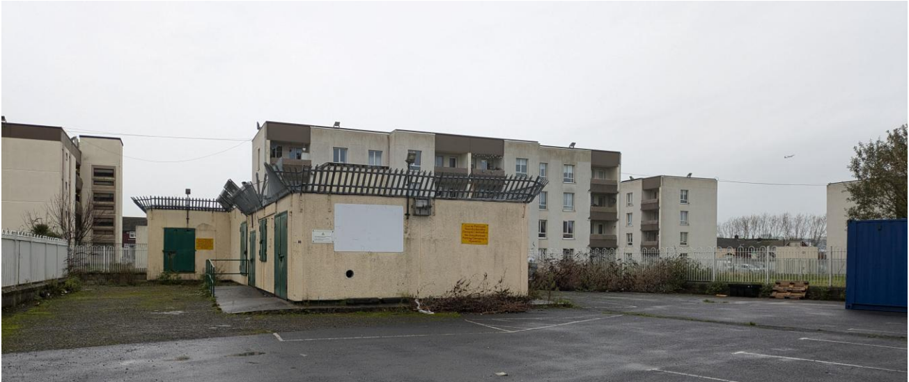
Figure 6: Single storey structure to be demolished
