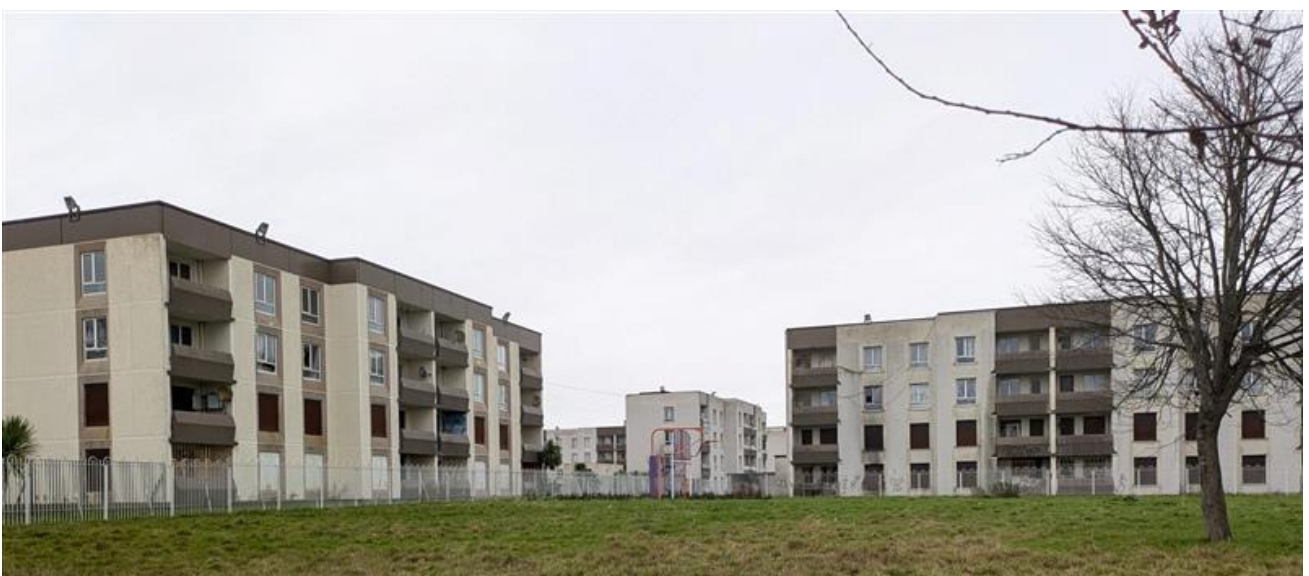
Figure 5: Vacated blocks to be demolished
