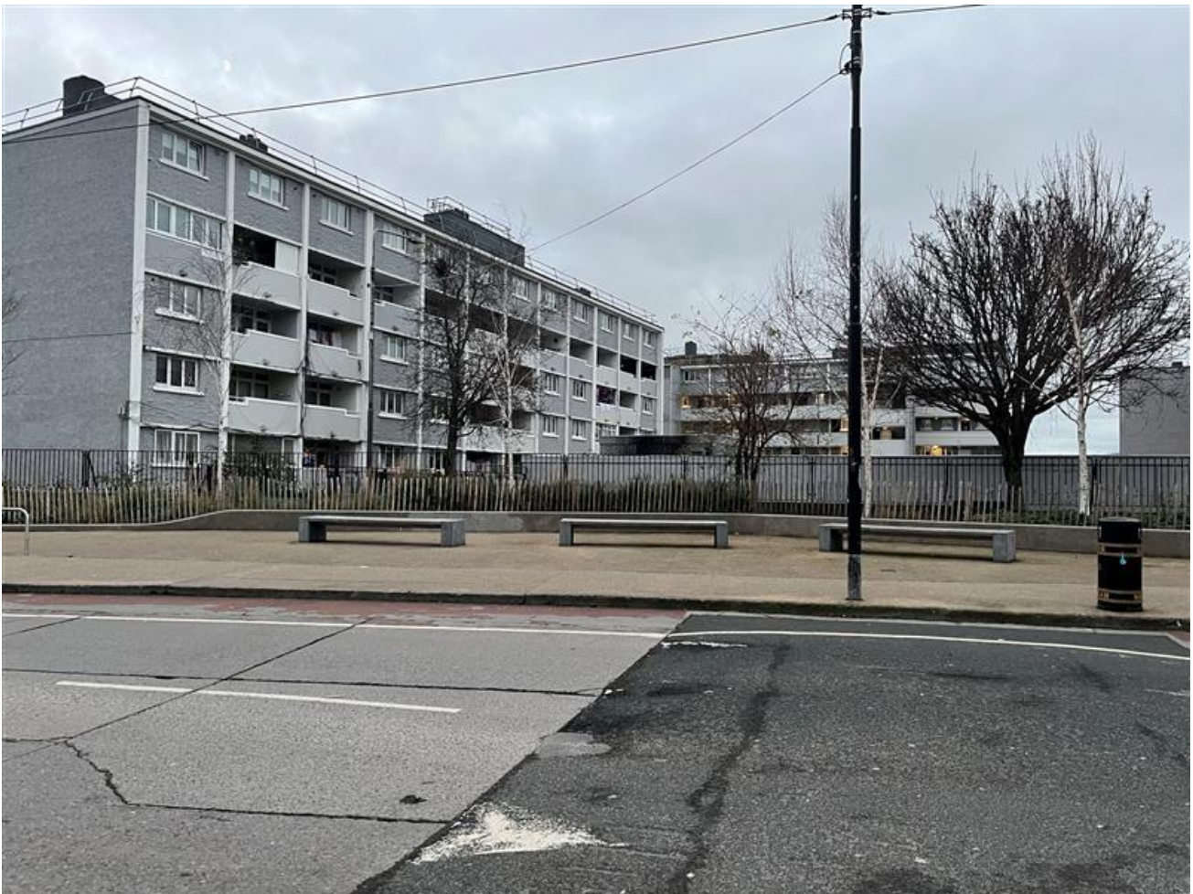
Figure 14: Public seating across from site (facing south-east)
