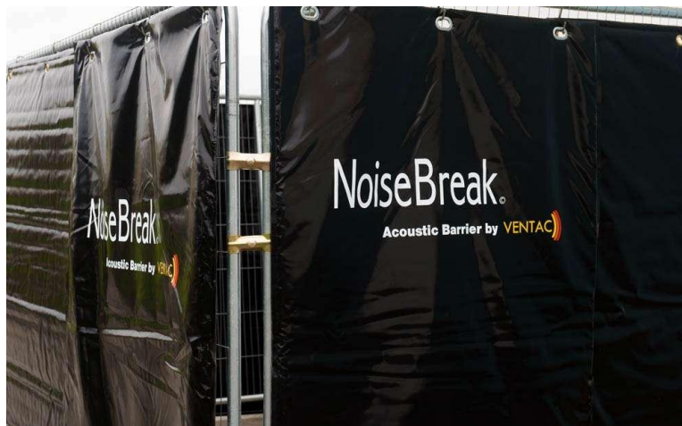
Figure 15: Temporary Construction Noise Barrier © Ventac
