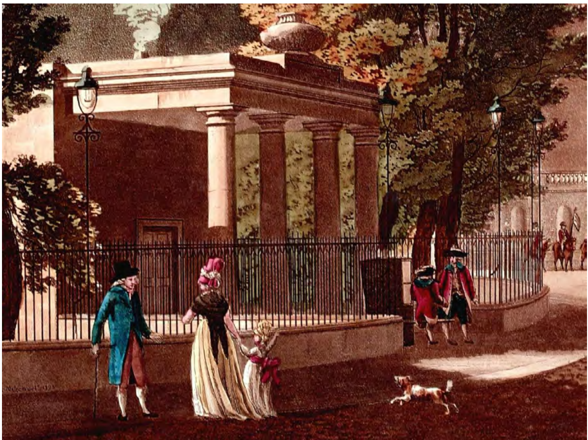
Fig. 15: Extract from James Malton's view of Rutland Square, c.1790s, showing the elegant array of lamp irons as newly erected on the railings that were installed as improvements carried out to the perimeter of the Rotunda gardens in 1784-85. This view is probably the best representation of modest railing-mounted lamp irons on a Dublin square and are directly comparable, perhaps minus scrolling ornament, to the original lamp irons of Mountjoy Square.
