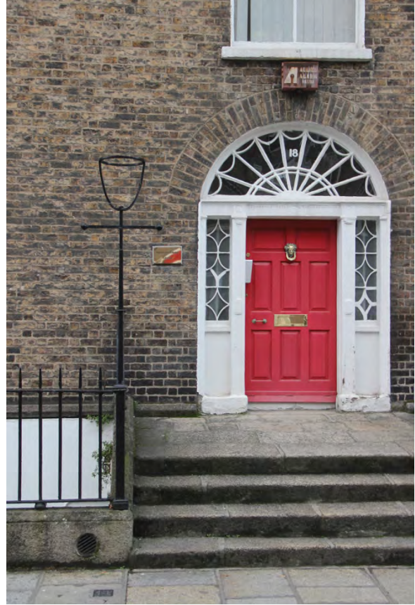
Fig. 27: Contextual view of lamp iron.
