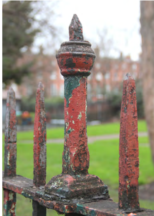
Fig. 34: Mountjoy Square former lamp iron Newel, shaved to a sharp point with collar.
