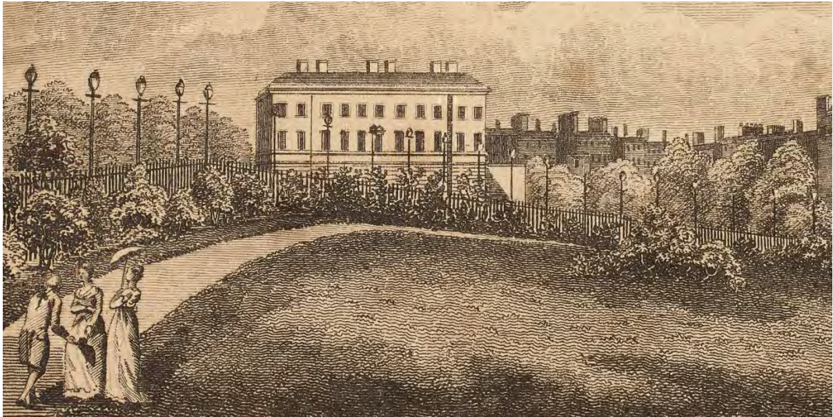
Fig. 18: View of Merrion Square and Leinster House showing the array of original railing-mounted lamp irons surrounding the west and south sides of the square.
