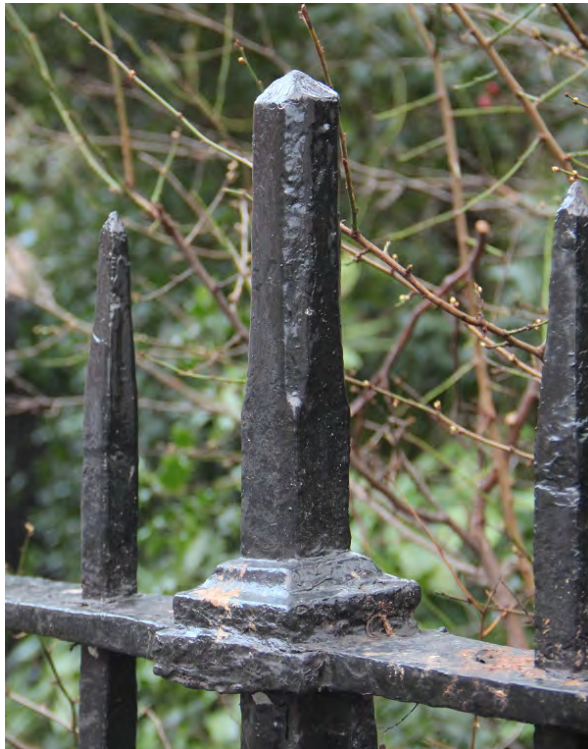
Fig. 33: Fitzwilliam Square former lamp iron newel, shaved to a blunt point.
