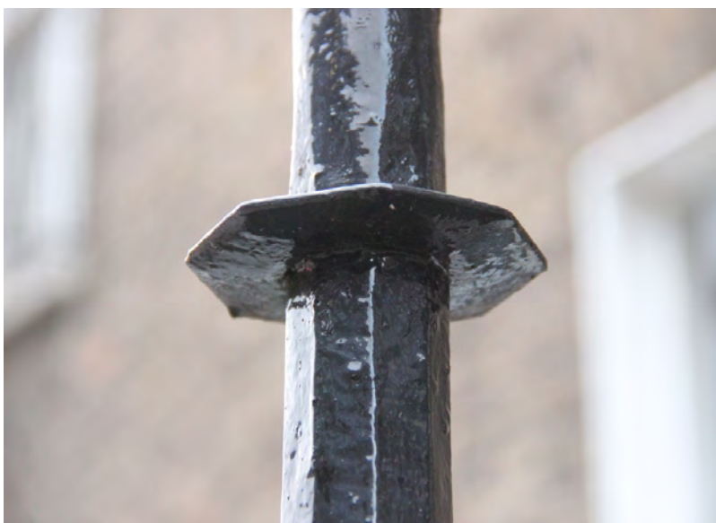
Fig. 28: Detail of profile transition from multi-sided base to rounded column.
