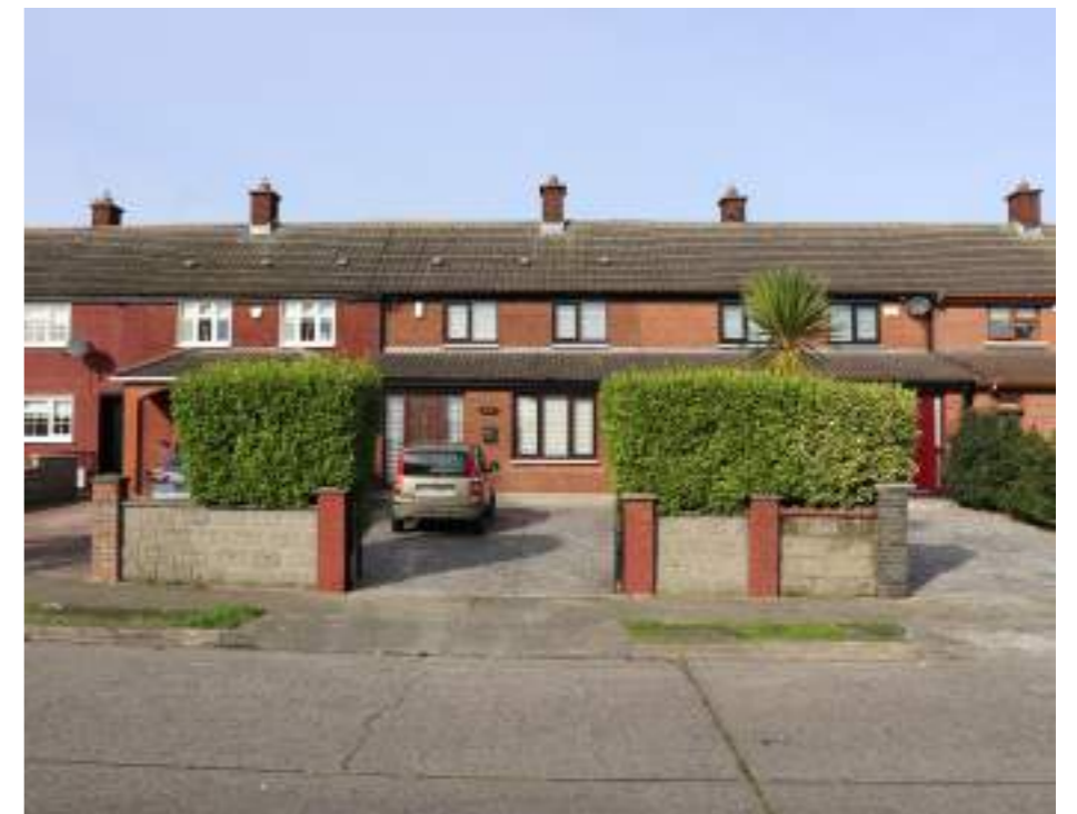
Terraced Houses on Cromcastle Park
