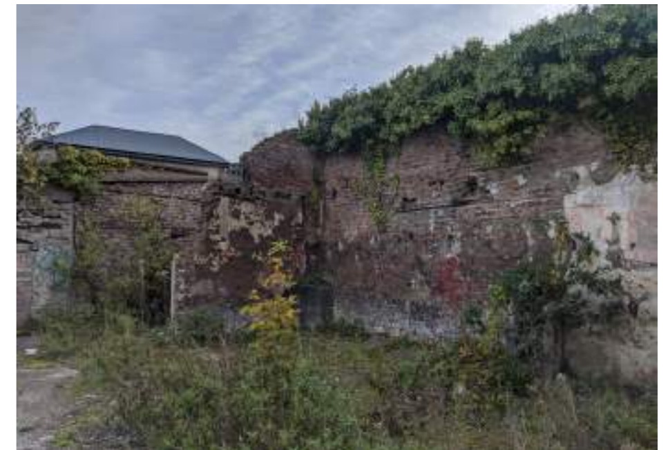
View towards Rear of Woodville House with Existing Walls in foreground
