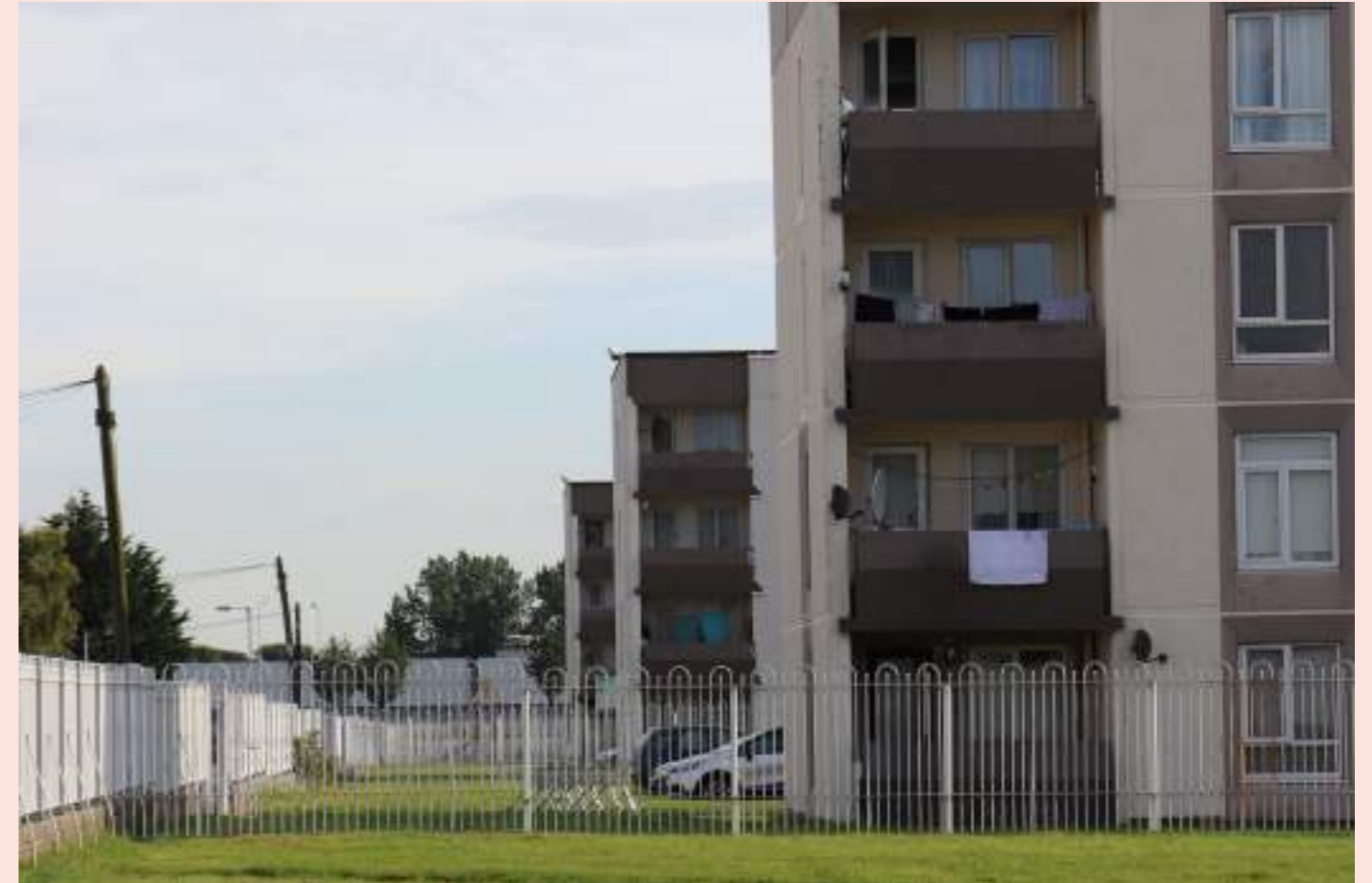
Cromcastle Court Estate, Existing Buildings
