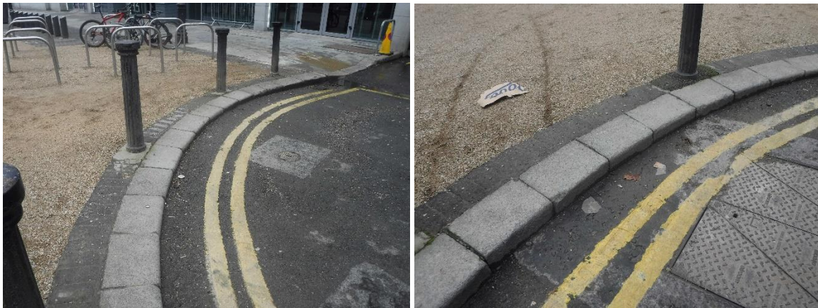
Figure 43 & 44 Photograph of historic Leinster granite kerb, Findlater Place.
