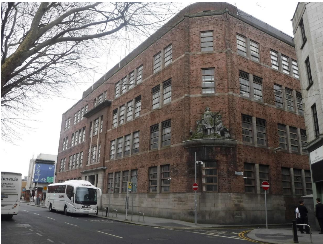
Figure 14 Streetscape photo of Cathal Brugha Street / 66-72 Marlborough Street, Dublin 1, Further Education Training College, looking west on Cathal Brugha Street.
