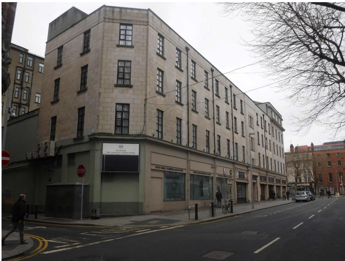
Figure 15 Streetscape photo of Gresham Hotel looking west on Cathal Brugha Street.
