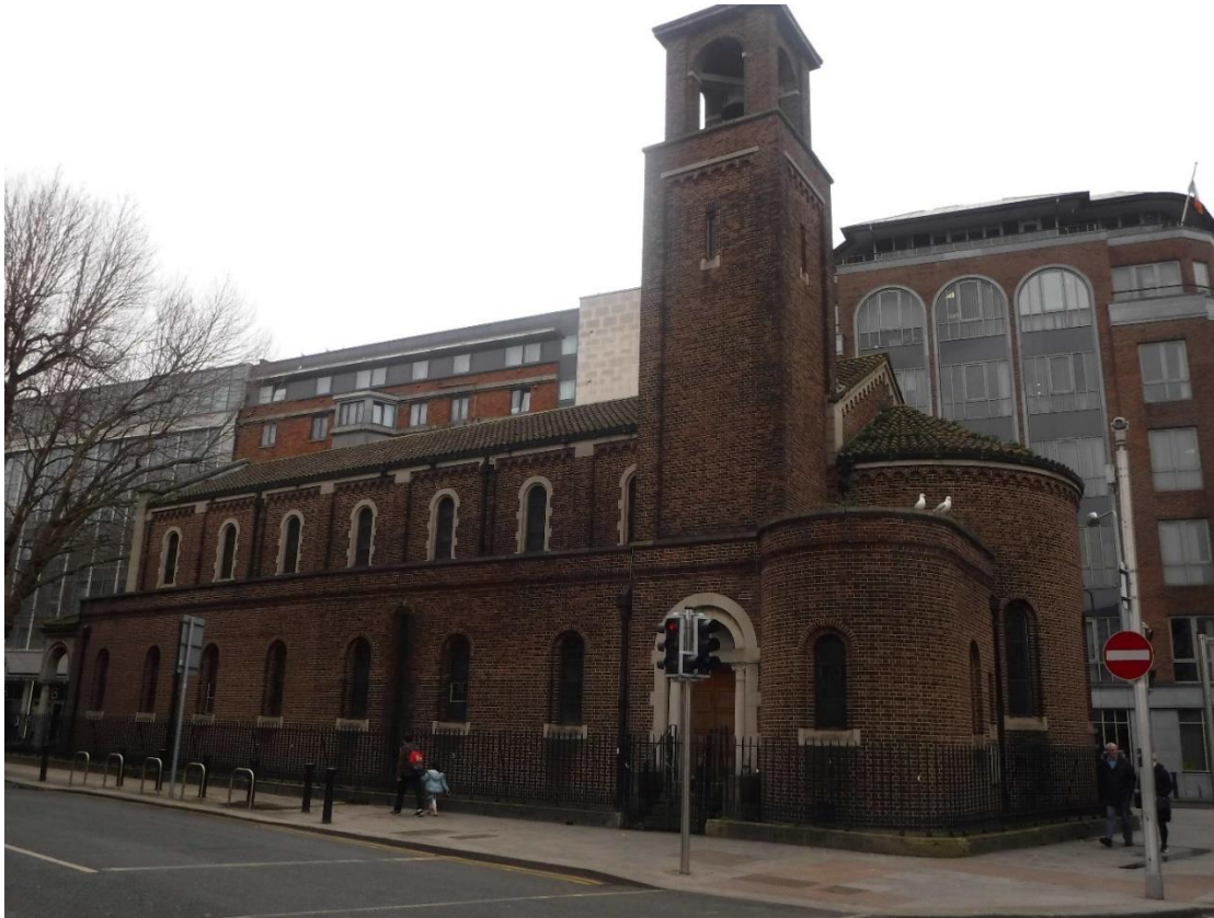
Figure 18 Streetscape photo of Saint George & Saint Thomas Church, looking west on Cathal Brugha Street.
