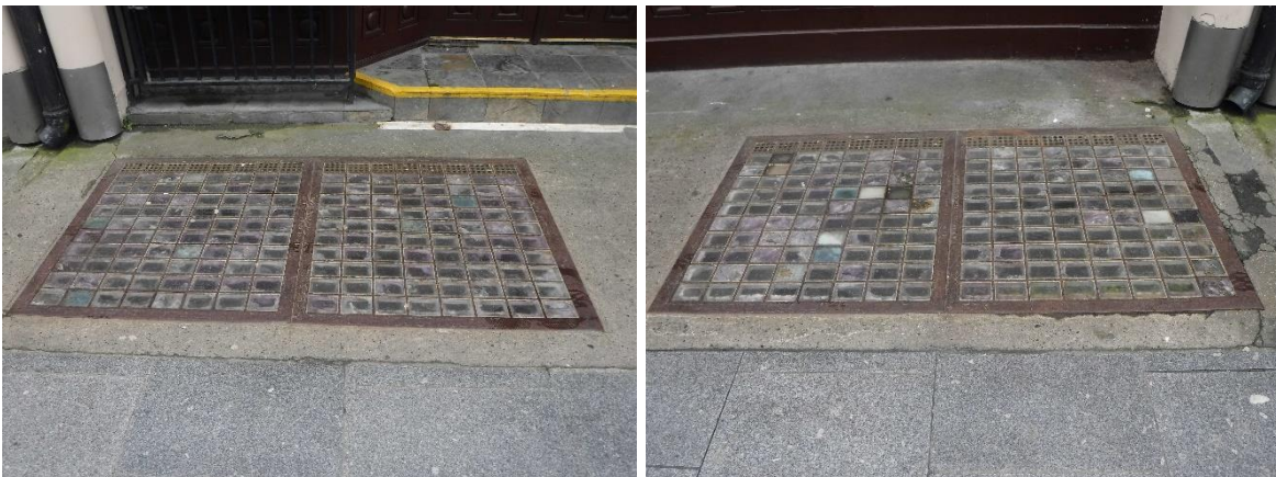
Figure 22 & 23: Photographs of cellar lights, Gresham Hotel, Cathal Brugha Street.
