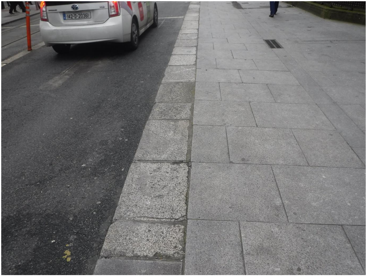
Figure 48 Photograph of heritage Leinster granite kerb, Marlborough Street.
