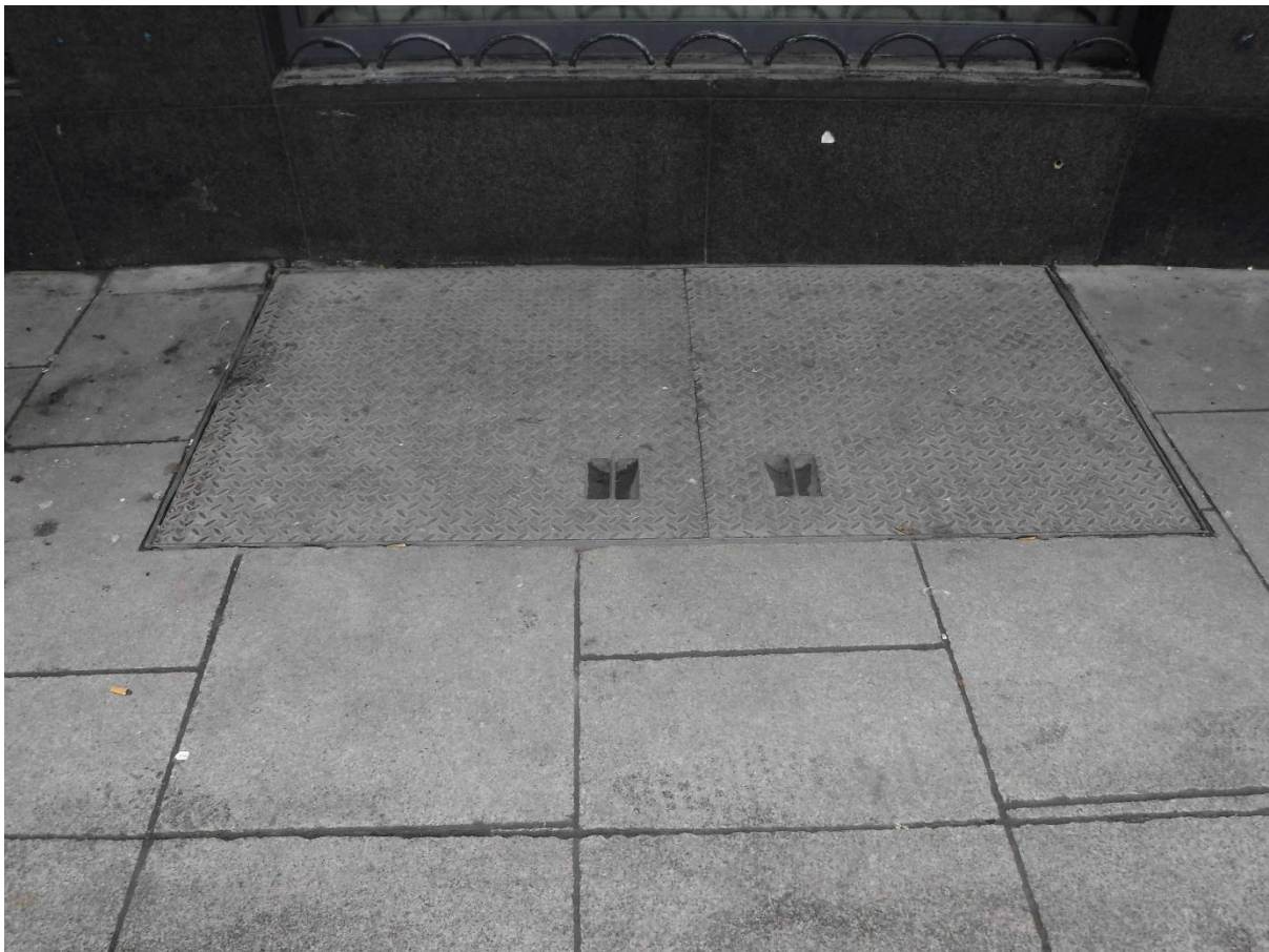
Figure 47 Photograph of modern cellar hatch, Findlater Place.
