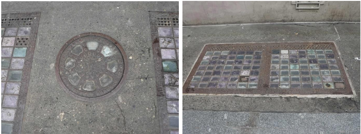
Figure 25 & 26 Photographs of cast iron access hatch and cellar/ basement lights, Gresham Hotel, Cathal Brugha Street.
