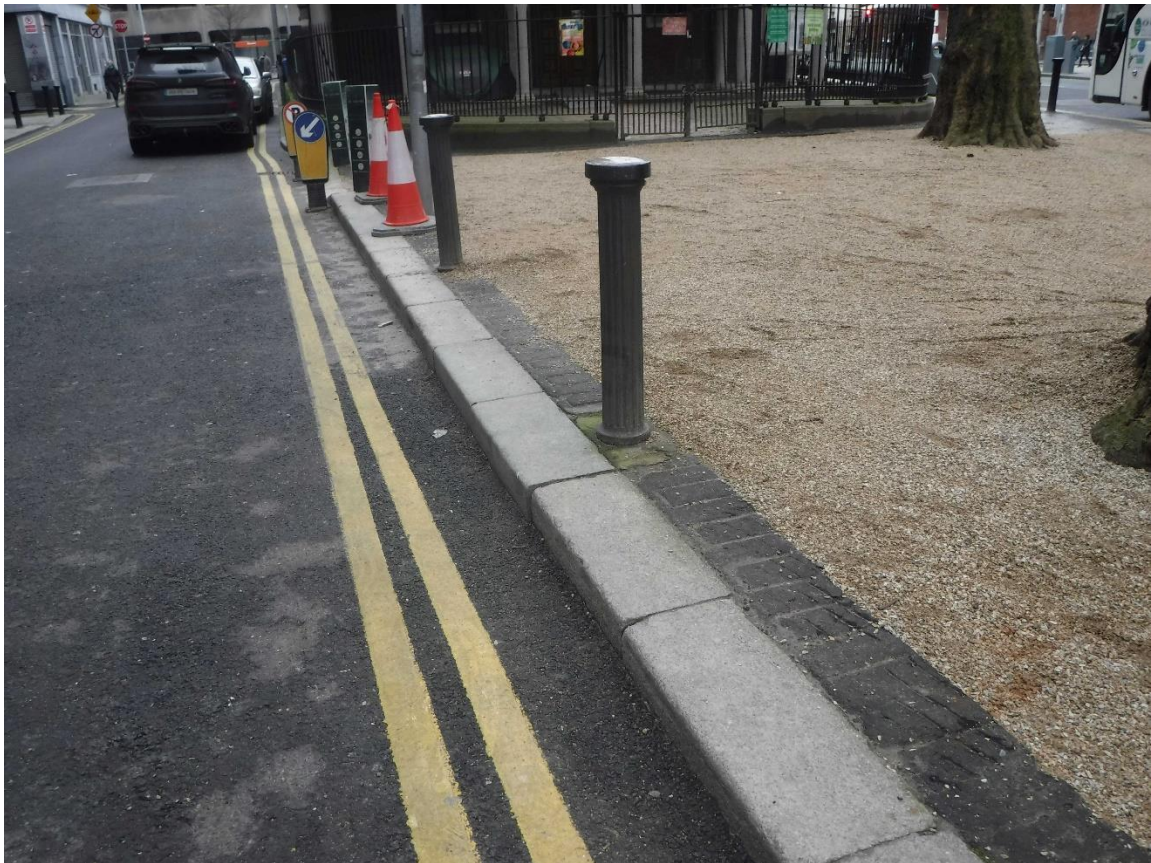
Figure 45 Photograph of historic Leinster granite kerb, Findlater Place.
