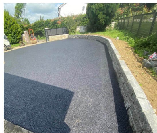
Tarmacadam with Pigmented Chippings to Homezones and Link Road
