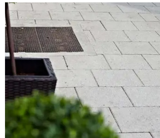
Concrete Flagstone Paving to Courtyard
