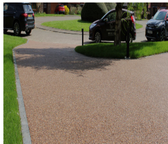
Resin Bound Gravel Surface
