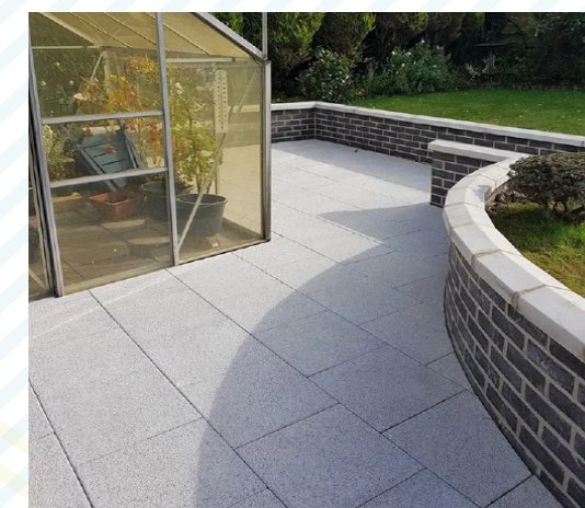
Concrete Pavers to Patios
