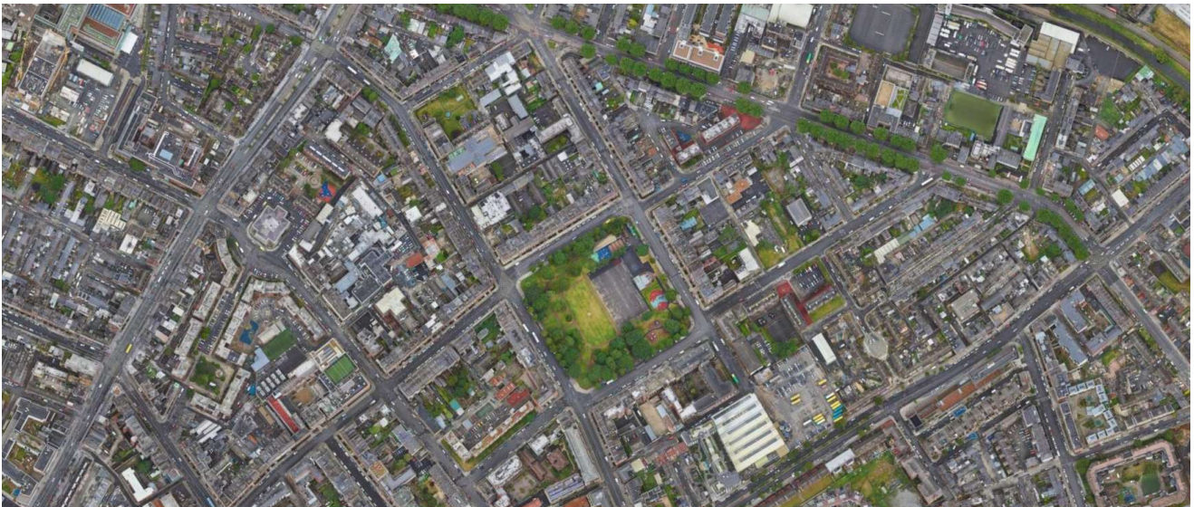
Figure 1. Aerial photograph of Merrion Square in north city centre Dublin context (imagery copyright 2025 Airbus, Maxar Technologies, Map data 2025)
