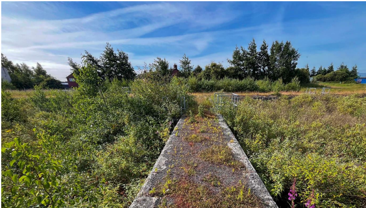
Fig 5. Overgrown Disused Water Storage Tanks at Bluebell Lands. 2024.
