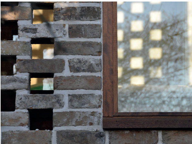
‘Hit and Miss’ Brick Detail, Grafton Architects: Waterloo Lane Mews House
