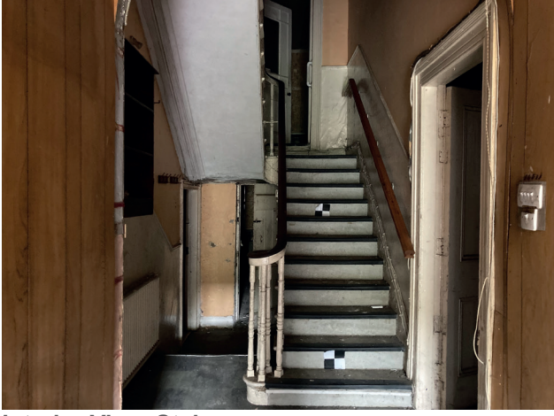
Interior View, Staircase
