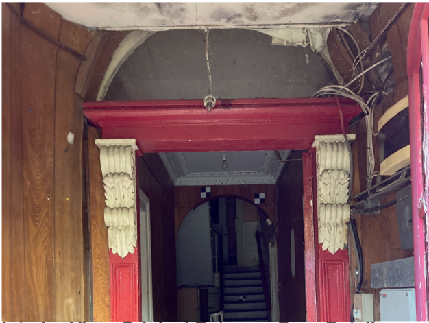
Interior View, Original Entrance Door Detail
