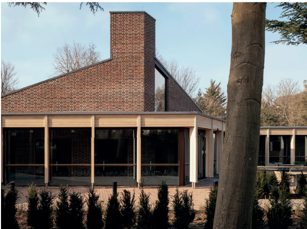
Timber Pergola, Mae Architects: Morden Centre
