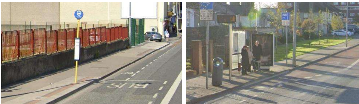
Figure 2-2: Left, Northbound Bus Stop and Right, Southbound Bus Stop on the R110 Dolphin's Barn Road
