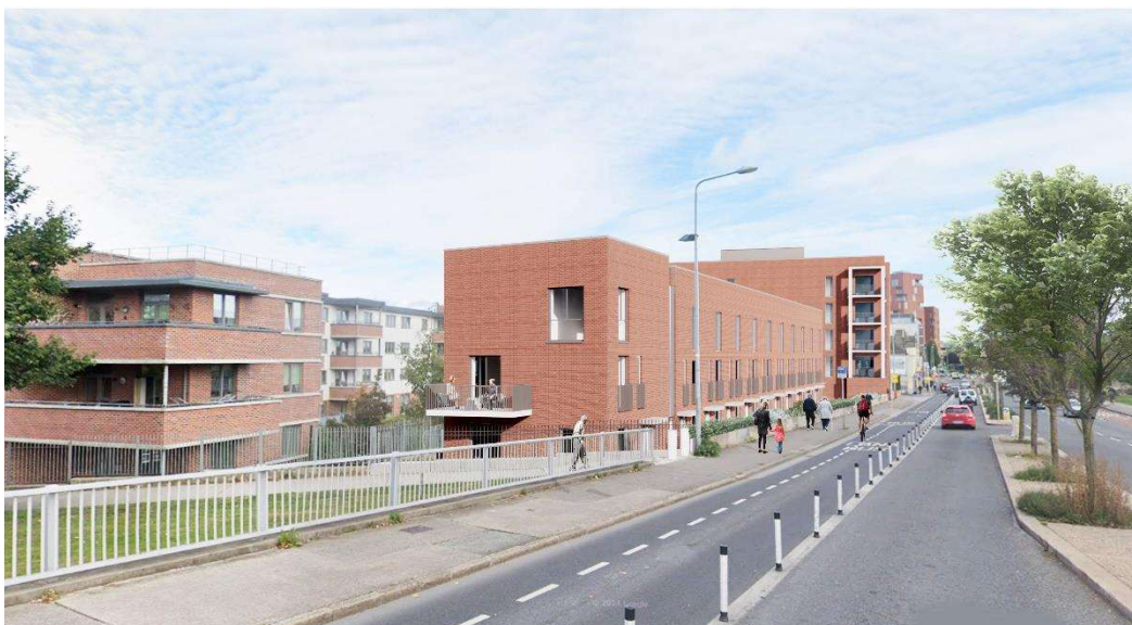
Figure 1-3: Perspective from R110 Dolphin's Barn Road
