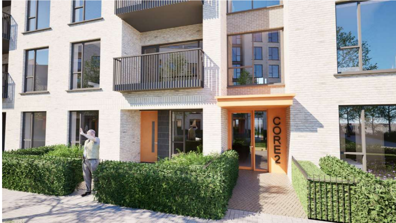
Image 63 - View of the typical ground floor treatment
