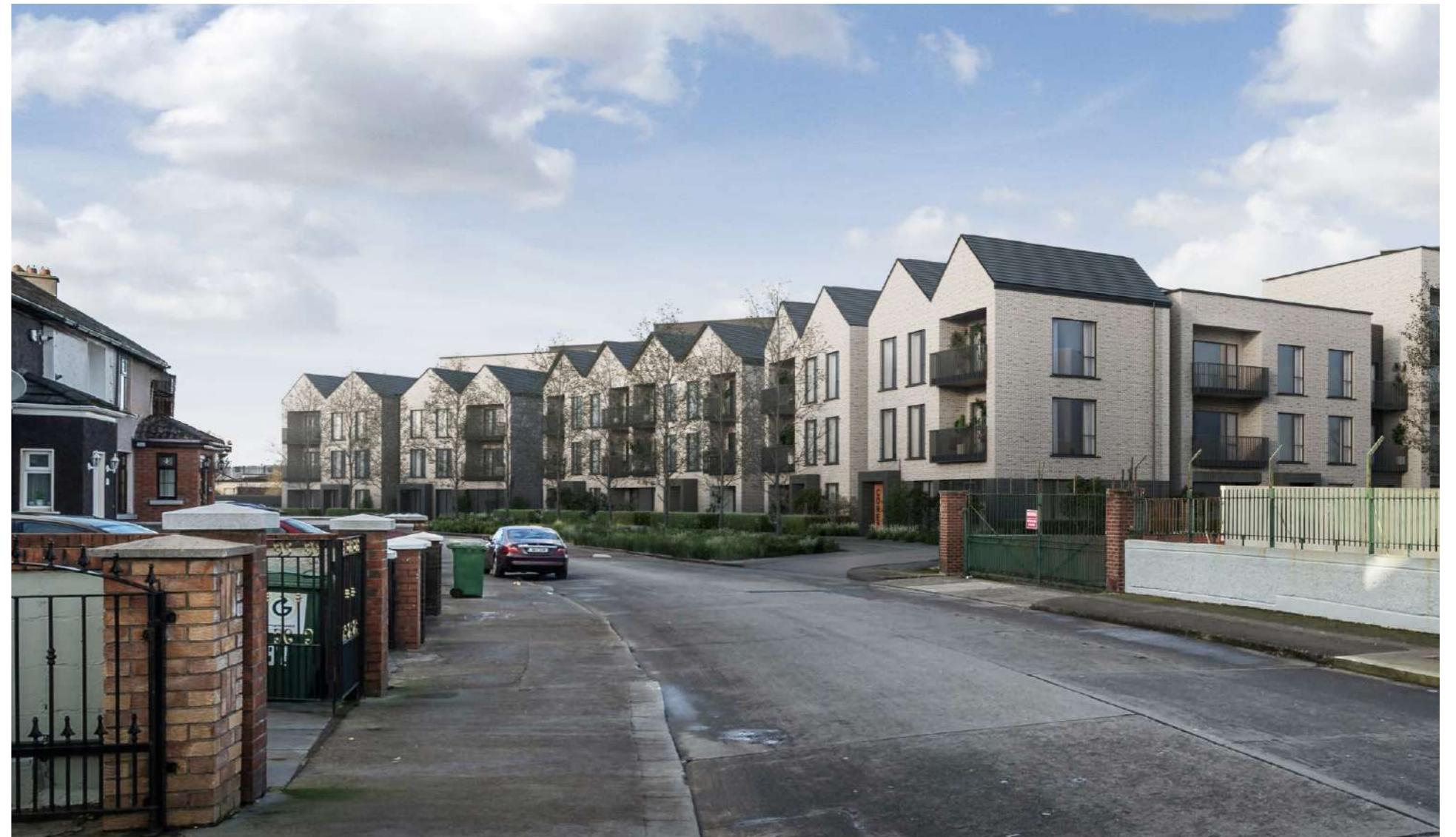
Image 38 - View of Bannow Road
