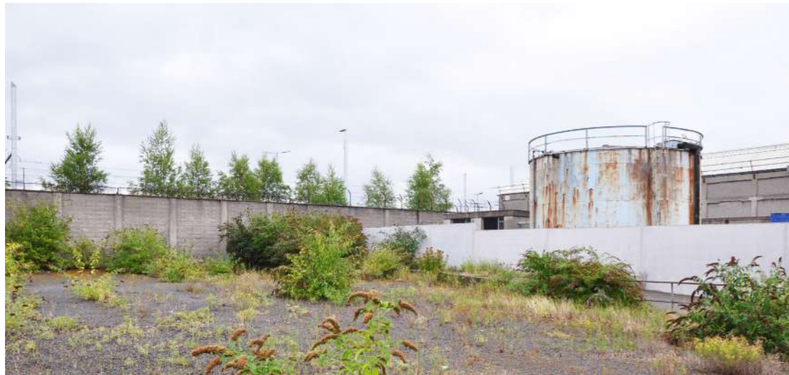
Image 12 - Existing block wall boundary to the railway line (left) and newer concrete wall boundary to Batchelors site with silo structure behind (right)
