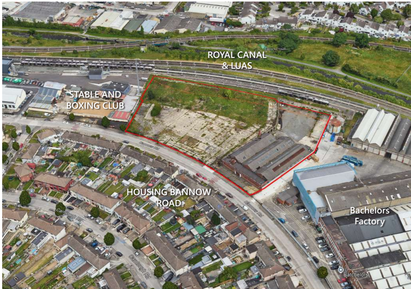
Image 18- Aerial 3d view of the site and surrounding buildings
