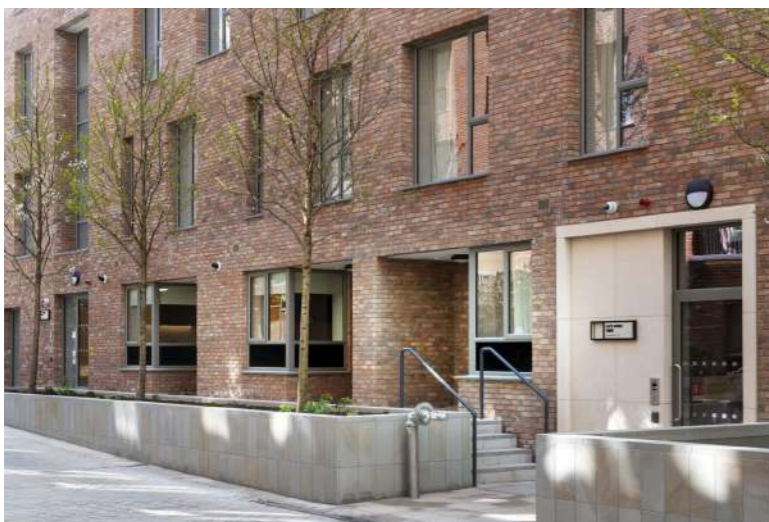
Image 47 - Charlemont Regeneration - MCORM Architects - own door units at ground level
