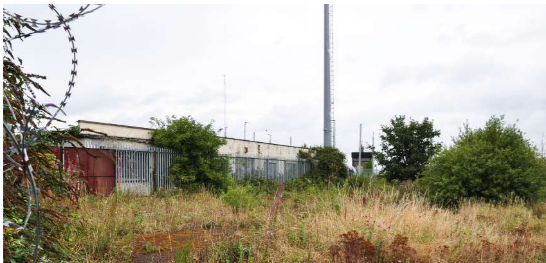
Image 13 - Palisade fence boundary to the Stables and Boxing Club site
