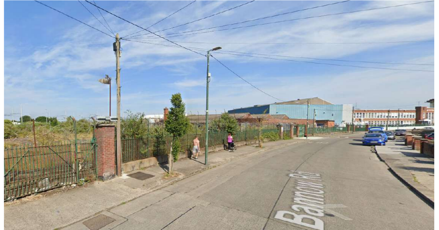
Image 14 - View of site frontage from the north on Bannow Road
