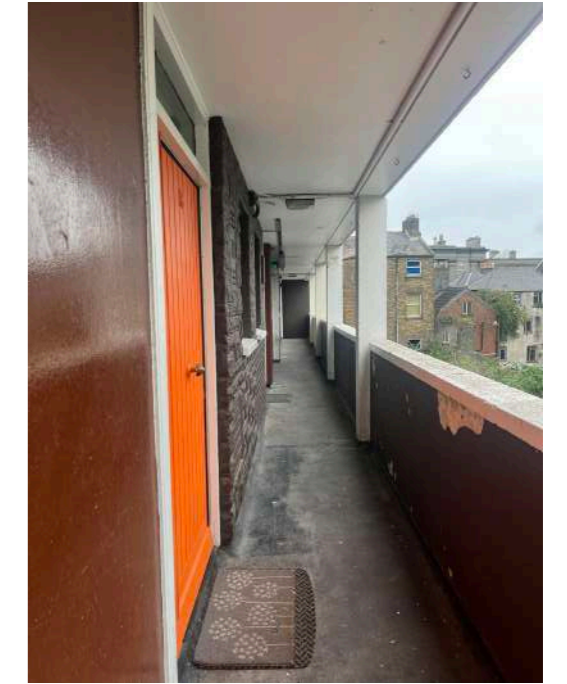
Typical upper external walkway (York Street block)
