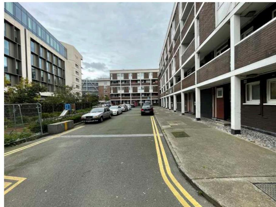
Courtyard view towards Mercer Street Block
