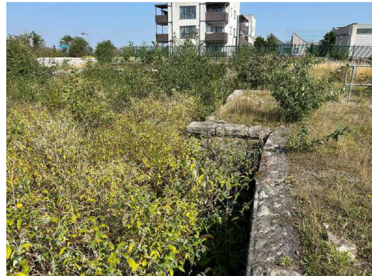
Plate 9: Detail of granite coping stones, facing east-northeast
