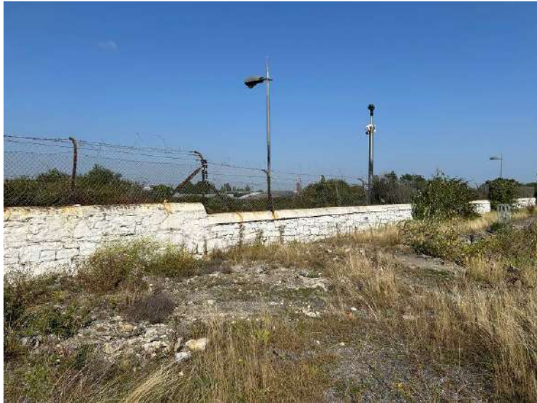
Plate 10: Northern boundary wall, facing northeast
