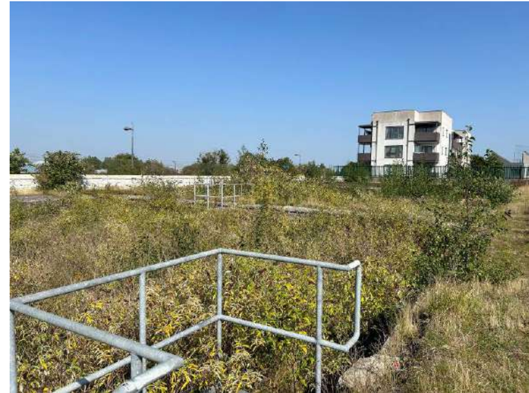
Plate 7: 19th century filter beds, facing east-northeast
