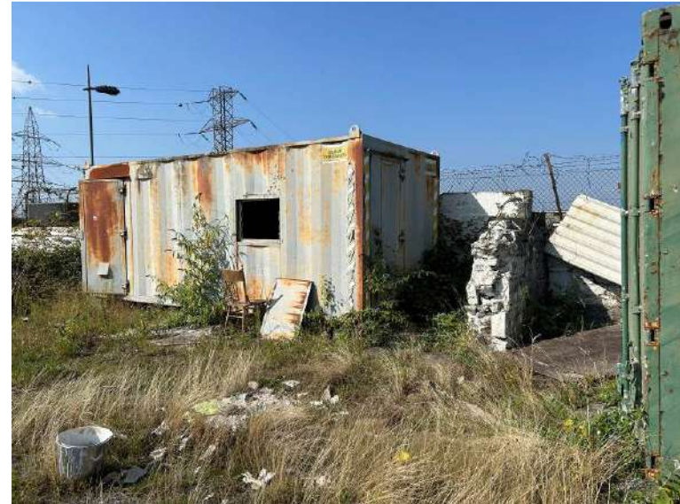
Plate 11: Return of screening wall associated with the Lock Cottage, facing northwest
